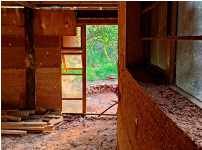
An example of a hempcrete wall
