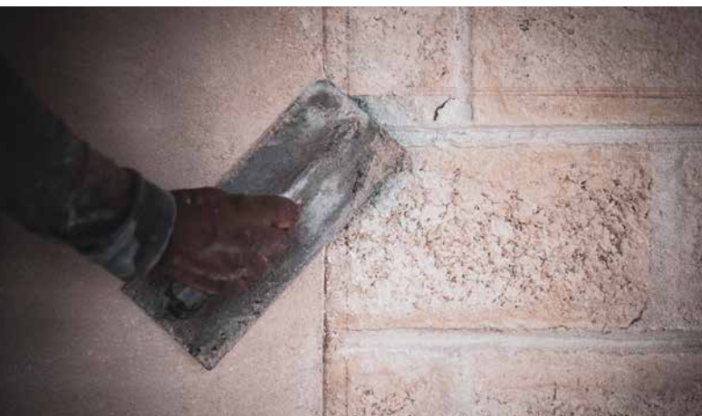
Hemp lime plaster and hempcrete blocks
